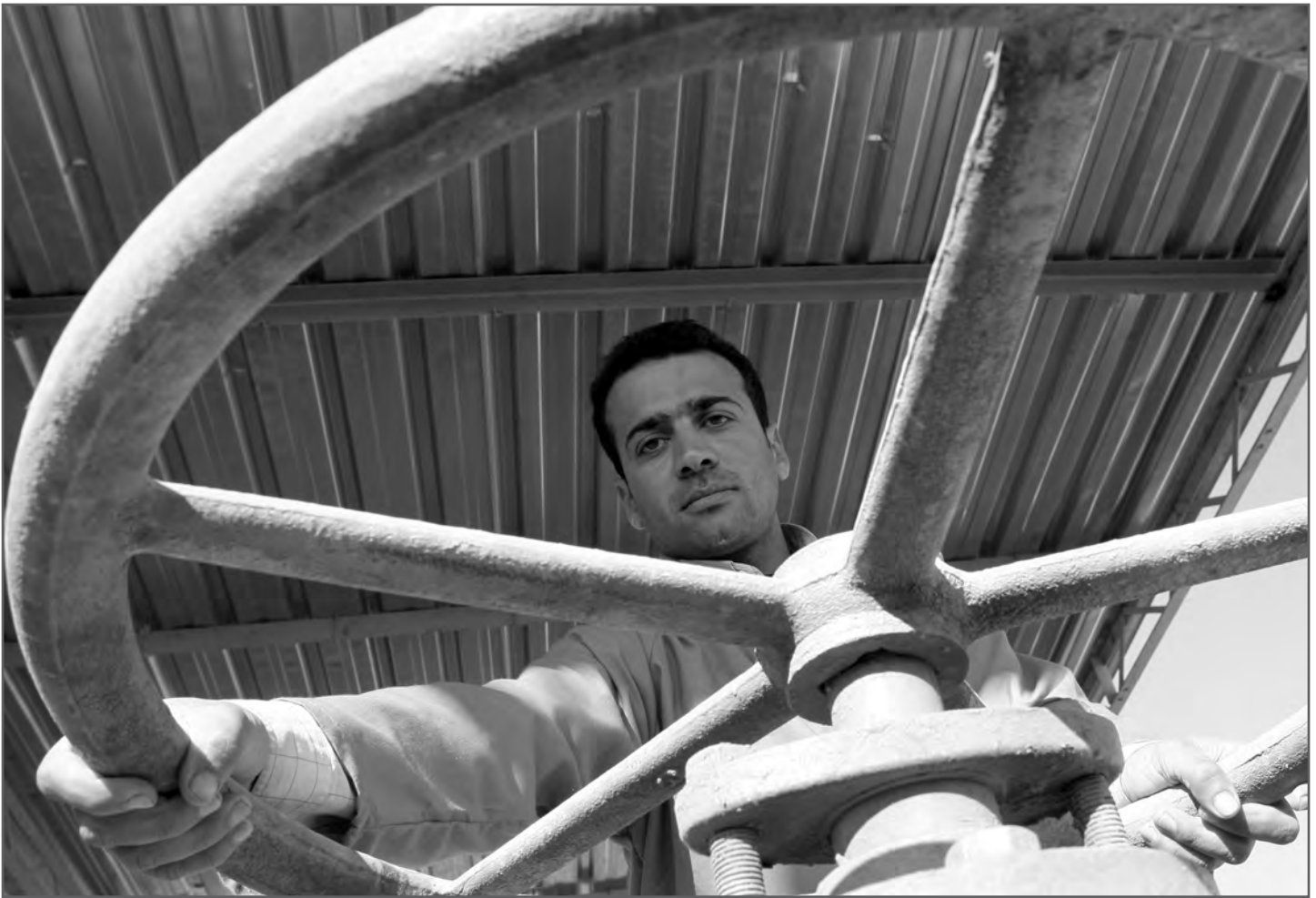
A man operates pipe infrastructure in Iraq. (Photo by UDAID/Iraq)
