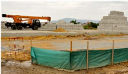
Completed CMU blocks stacked at site (Photo: R. Nyberg, USAID)
