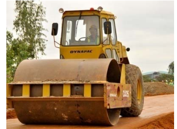
Compacting fill material (Photo: R. Nyberg, USAID)
