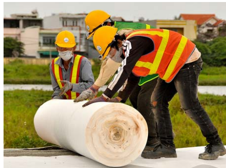
Installing the liner of the drying pad foundation (Photo: R. Nyberg, USAID)
