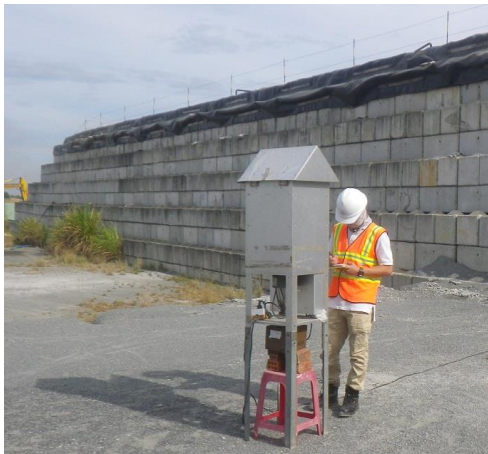
Air sampling at the perimeter of the treatment structure during quenching. (Photo: CDM Smith)
