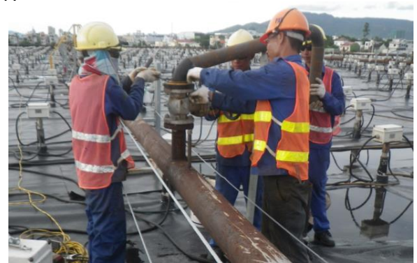
Installing the vapor extraction manifold on top of the thermal treatment structure for Phase 2 (above)
