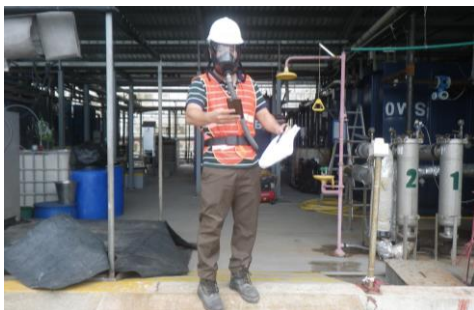
Wearing appropriate PPE inside the liquid-vapor treatment plant while preparing and inspecting the plant for Phase 2 thermal operations (Photo: CDM Smith)
