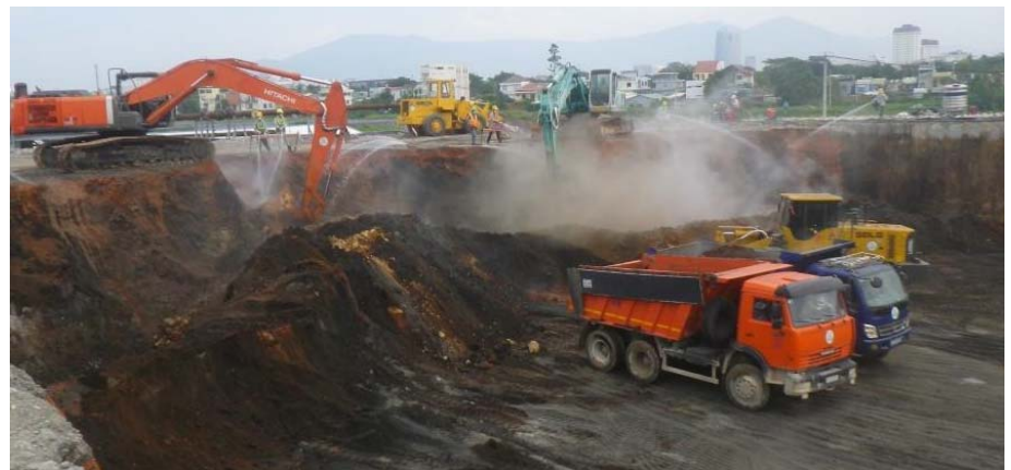
Removing Phase 1 treated soil and sediment from the thermal treatment structure
