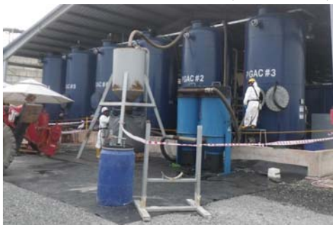
Removing spent carbon from the treatment plant
