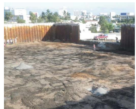
Inside the empty thermal treatment structure
