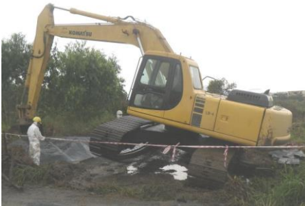
Decontaminating an excavator (Photo: CDM Smith)
