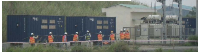
Installing power cables
