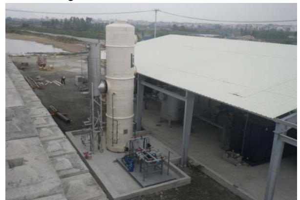
Liquid/vapor treatment plant construction (Photo: CDM Smith)
