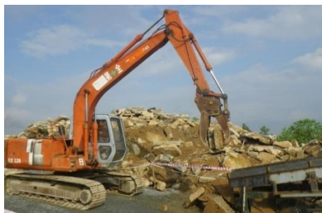
Cleaning and preparing concrete for crushing
