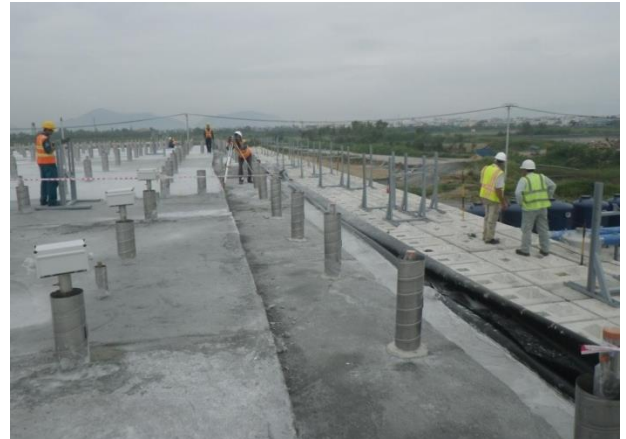
Concrete cap on containment structure (Photo: CDM Smith)
