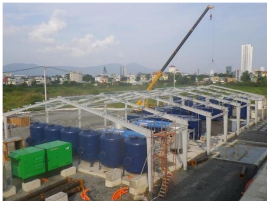
Liquid/vapor treatment plant construction
