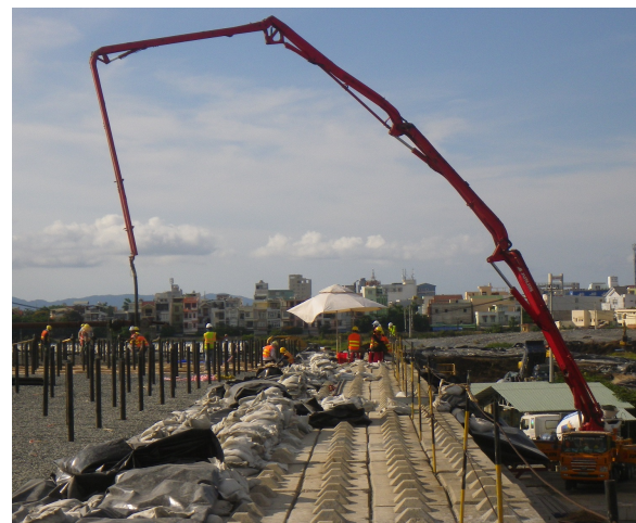
Installing heaters into the thermal treatment structure (Photo: CDM Smith)
