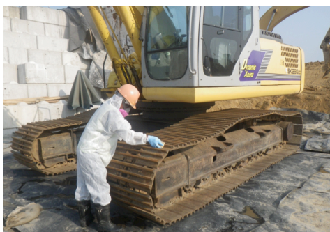
Decontaminating equipment (Photo: CDM Smith)
