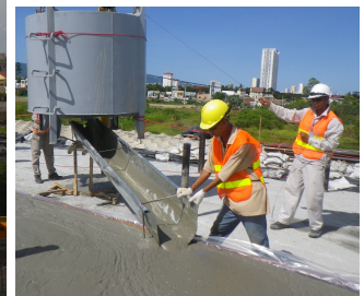
Pouring concrete layers on top of structure (Photos: CDM Smith)
