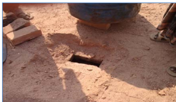
Figure 3.3 Hollow Space for fire and air movement. There is 3"-4" hollow space in between the column and the row and also in between two chambers for fire and air movement.
